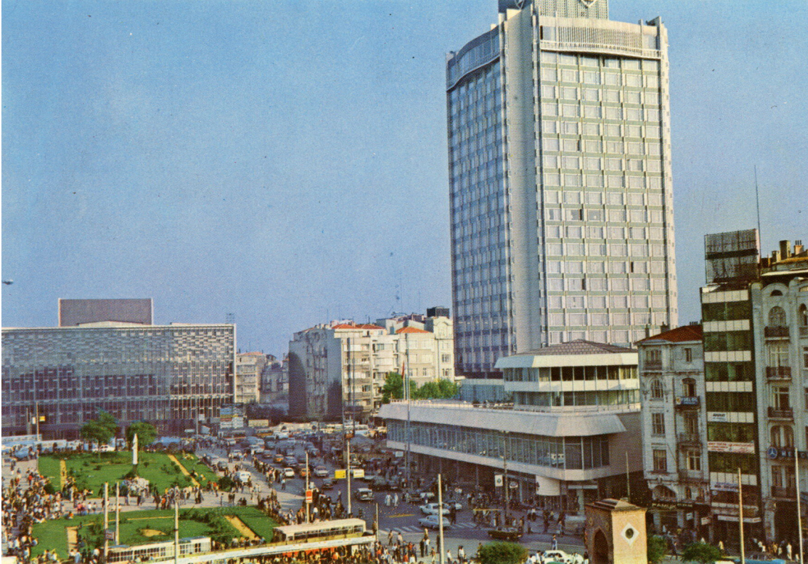
Figure 51: Etap Marmara Hotel
